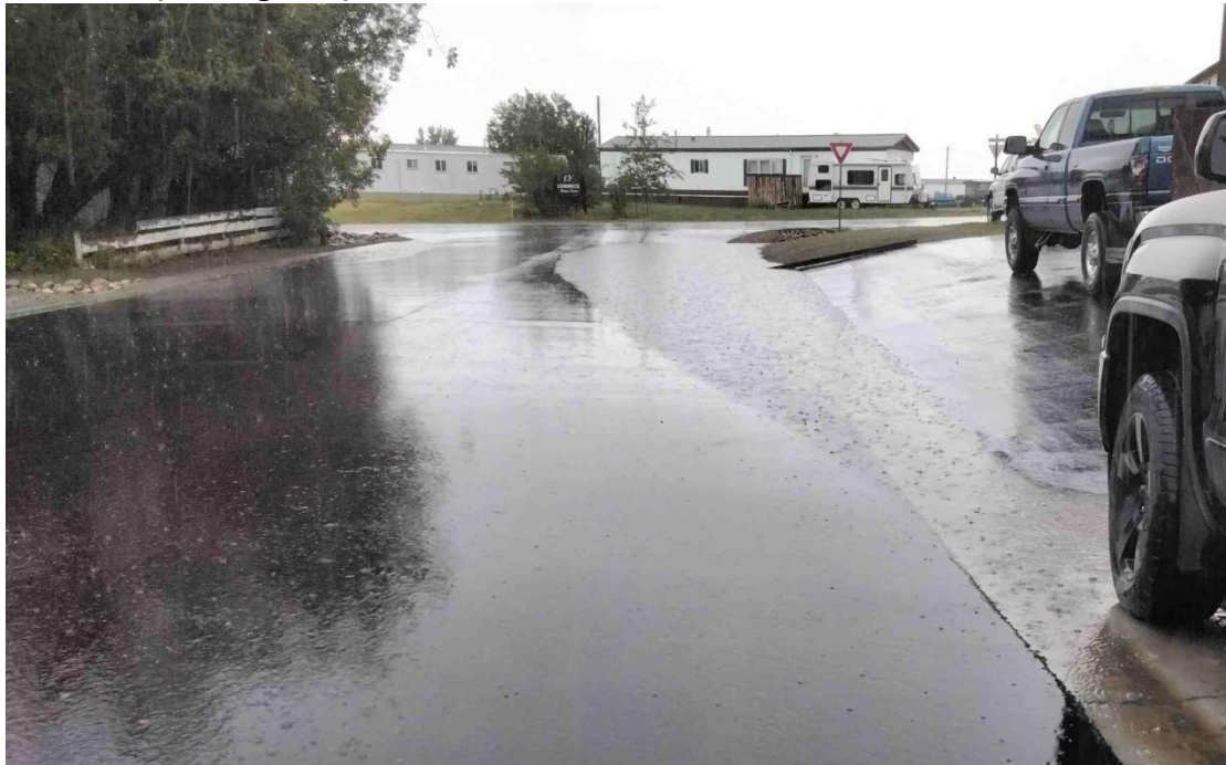
2 nd Street (looking east) water cannot traverse the crown
